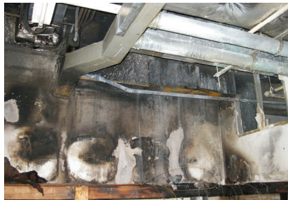
Basement Ceiling - Terminal Building
