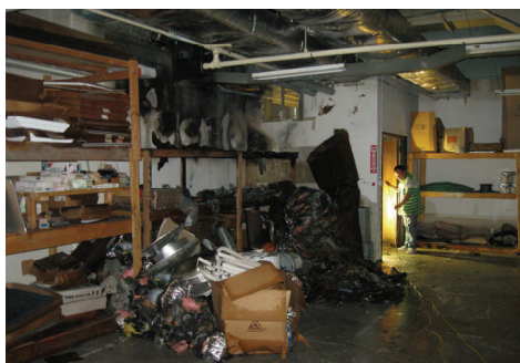
Basement Storage - Terminal Building
