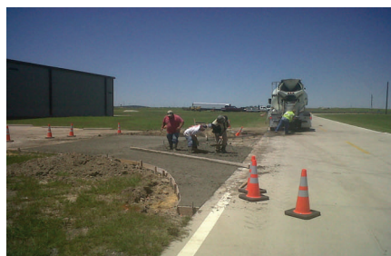
Driveway Installation - Spinks Airport
