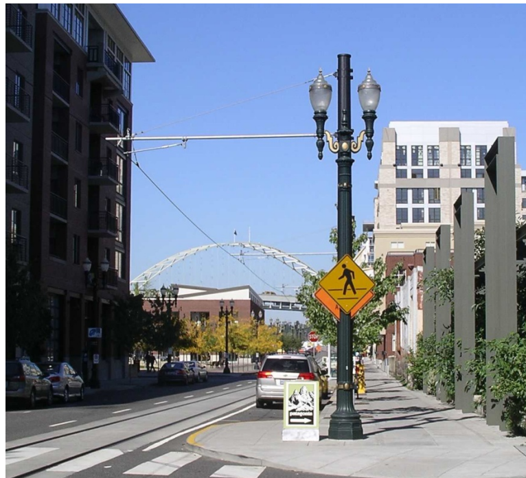
Fig. 8 – Trolley wire suspended by cantilever
