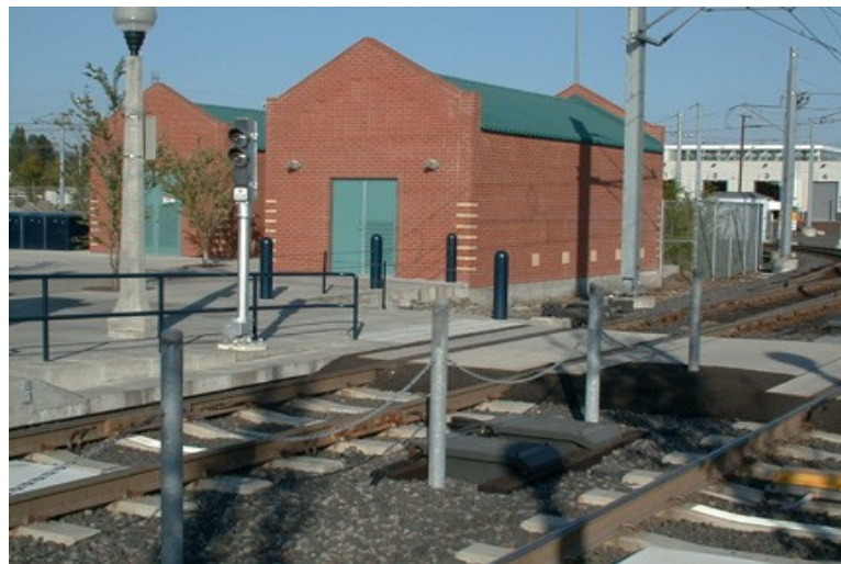
Fig. 4 – Building for High Power Substation
