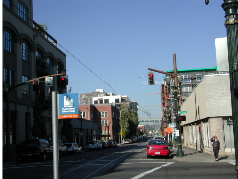
Fig. 10 – Span wires support by traffic signal poles
