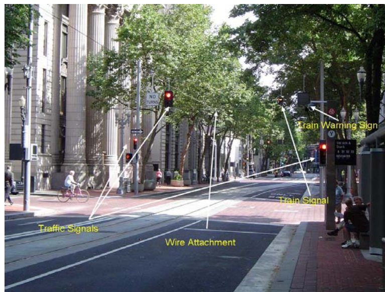
Fig. 13 – Traffic signal interface
