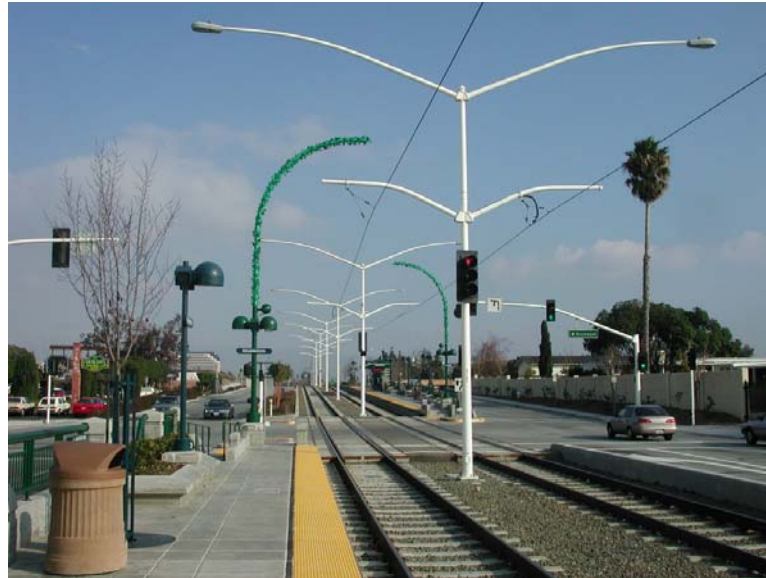
Fig. 9 – Joint use pole with Cobra heads
