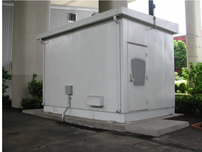
Figure 3 – Low Power Pre-fabricated Enclosure
